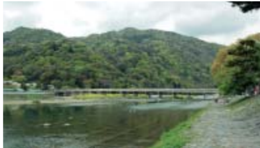
Togetsu-kyo Bridge in Arashiyama
